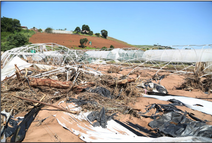
Shade net tunnels that were completely destroyed in the floods.
